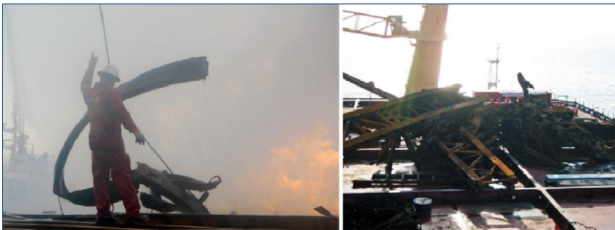
Figure 121—Debris removal activities on the platform
