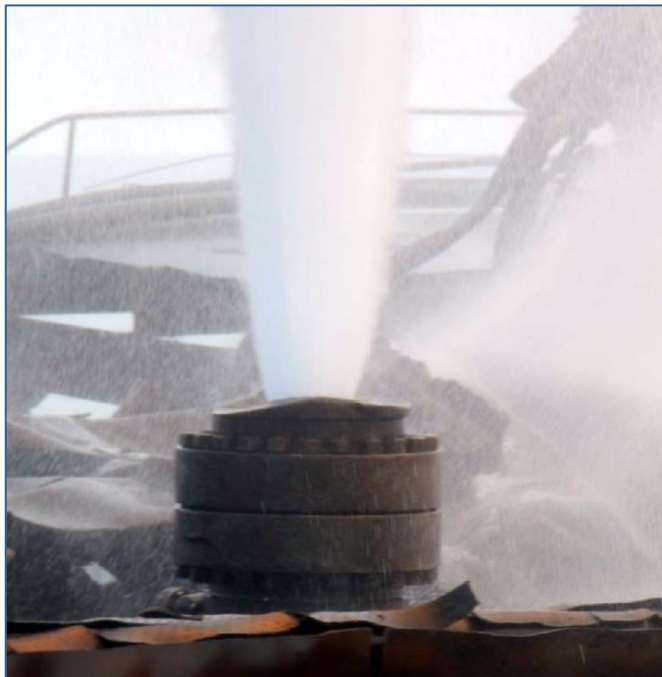
Figure 124—Unrestricted and vertical flow of the gas after cutting the wellhead
