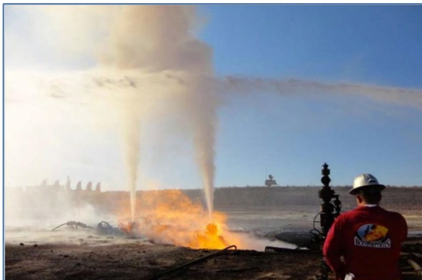
Figure 125—Cross-fire from failed wellheads intensified the operation complexity
